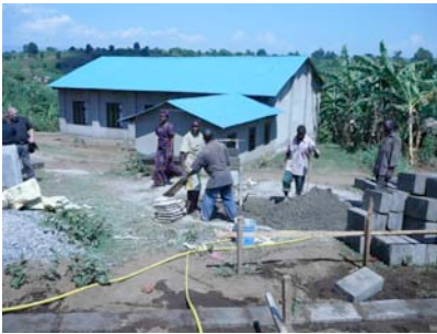
Work on Hostel with Mpuguso Lutheran Church in background
