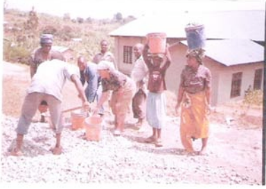
Working on the substructure
