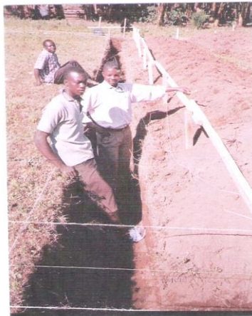
Digging the foundation
