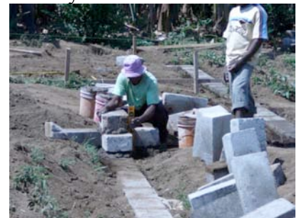
Laying Bricks at the future Hostel
